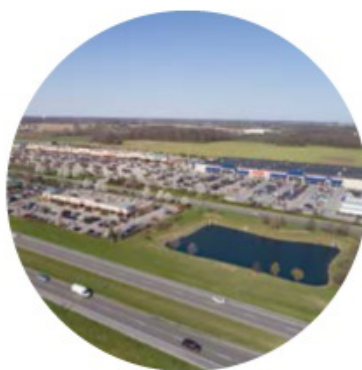
Emira Property Fund's Stony Creek Marketplace in Noblesville, Indiana, in the US
